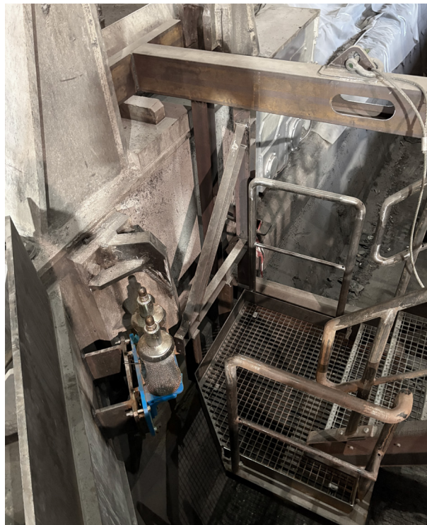
Image 4: Installation of couplerG on Ladle Car.
