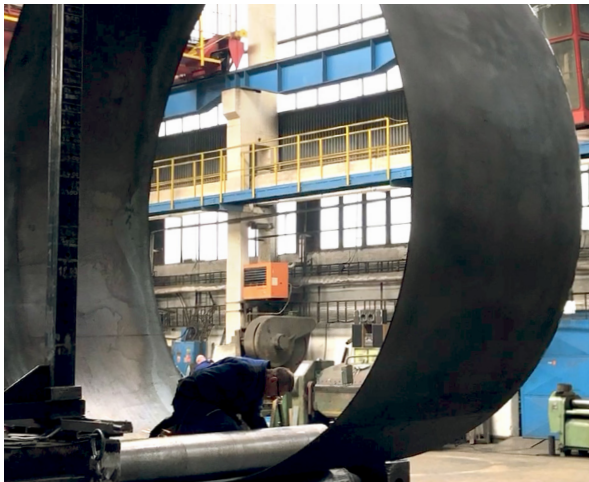
Figure 4: Step by Step. From the First Section Welding to the 250m³ Silo Complete Assembly.
