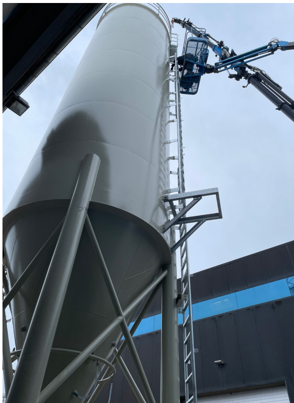
Figure 5: Installation at Site. Additive Silo 90m 3
