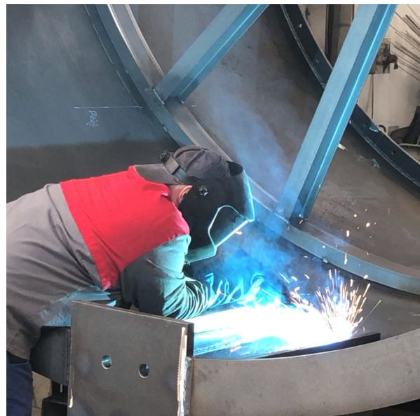
Figure 3: Precision Welding for Durable Silo Construction
